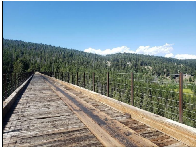
Figure 3 Thompson Park Trestle, Silver Bow County
