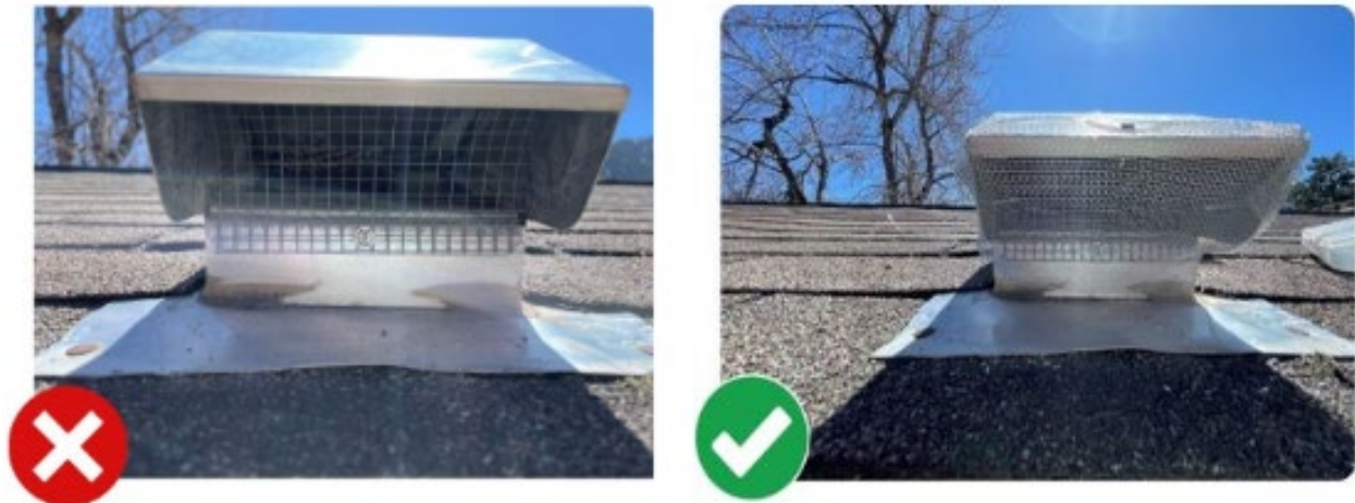
Figure 6.4. Examples of a bad vent (left) with 1/4-inch mesh that is ineffective at preventing ember incursion, and a good vent (right) that has 1/8-inch mesh to help prevent embers from entering the home.
