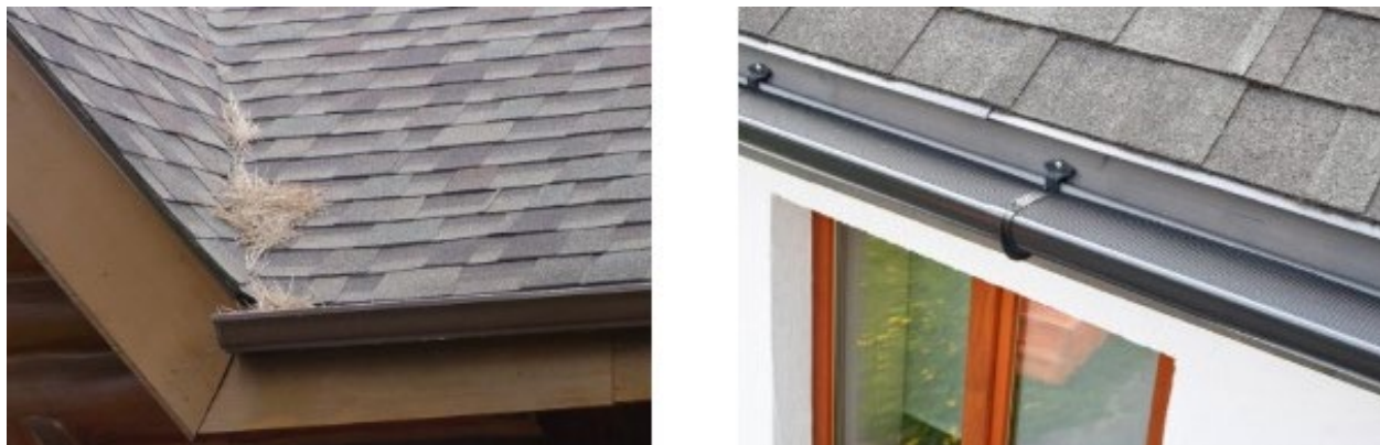
Figure 6.3. Examples of an uncovered gutter at risk of ignition (left) due to flammable tree debris, and a less-ignitable gutter (right) with a noncombustible gutter guard.
