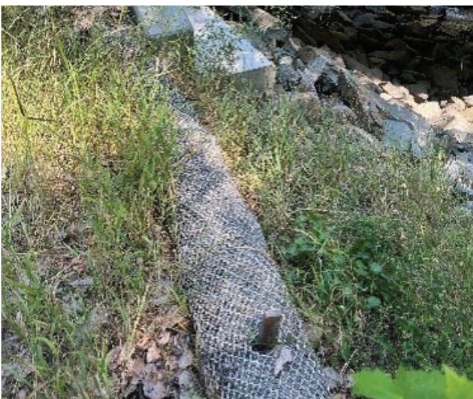
Temporary erosion control near a stream crossing
