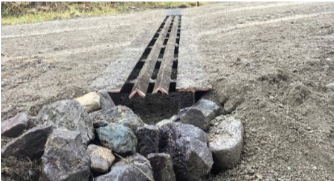
Drainage installation frequency to minimize erosion, reduce maintenance costs and protect water quality.
