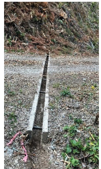
A maintained surface drainage feature
