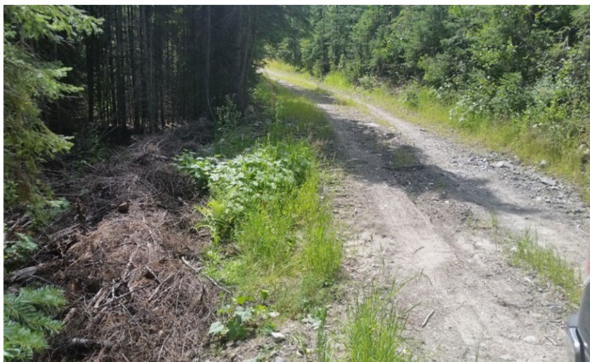
Photo 6: A slash filter used next to a road to provide filtration of runoff.
