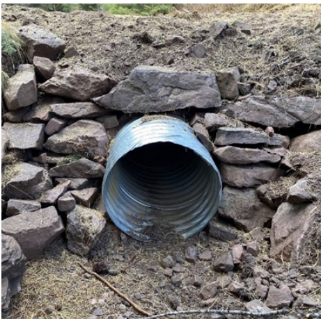
Photo 2: This picture is a good example of culvert that was design relief culverts with adequate length to allow for road fill width. This shows compliance to BMP III.C.3.
