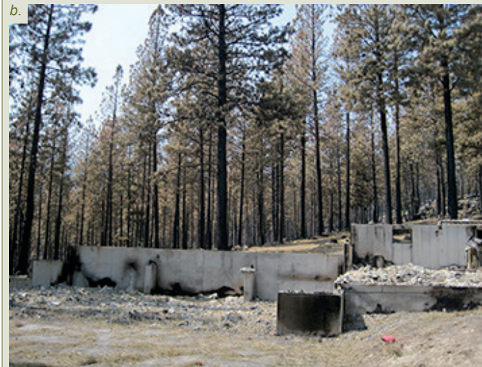
Figure 5. Two different houses a) and b). Neither house had adjacent high intensity burning. The charred and partially consumed trees adjacent to the houses burned from the burning house. The a) house did not have forest fuel treatment; the b) house had forest fuel treatment.
