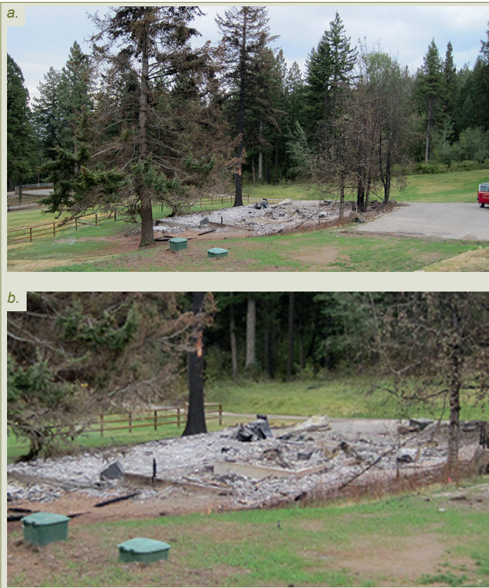
Figure 7. a) A wider view of the destroyed structure and surroundings. b) A narrower view detailing the surroundings. The destroyed structure is surrounded by unburned grass and unconsumed trees. The immediately adjacent trees were scorched and charred by the burning structure.
