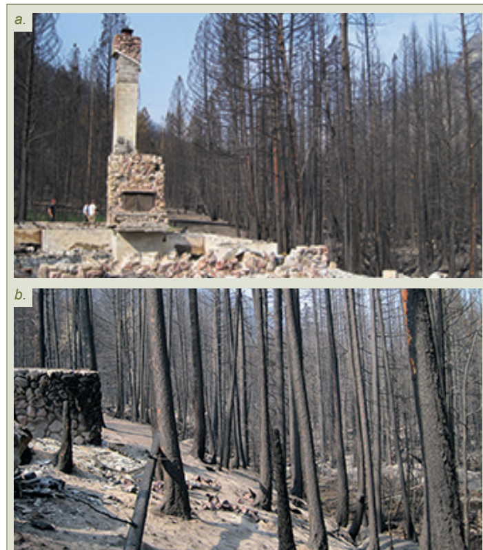
Figure 2. ACTIVE CROWN FIRE. These two separate but associated houses, a) and b) were several hundred feet apart. Both of these structures were 30 feet or closer to active crown fire.
