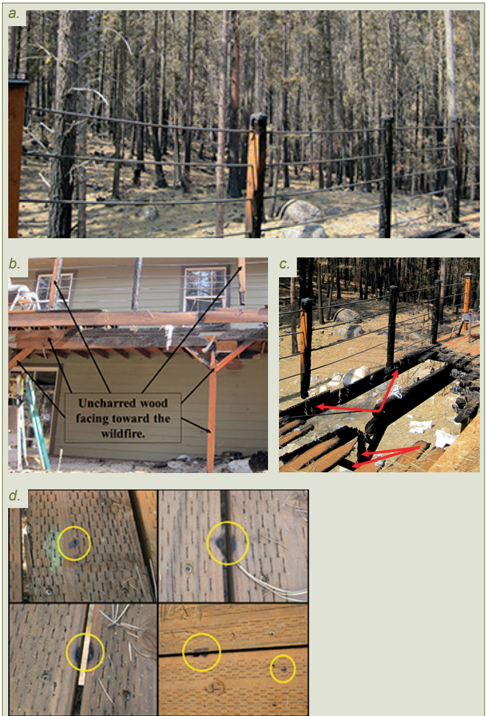
Figure 8. a) View from the burned deck at where surface fire spread to the house. No canopy fire occurred in the area immediately surrounding the house. Forest thinning and fuel treatment had not been done. b) Uncharred deck members on the sides facing the wildfire (black arrows). c) View of a portion of the burned deck (sheet of OSB covers burned-out gap in the lower right corner). The facing board and deck post sides are charred and had been burning (red arrows). d) Examples of the many firebrand char marks on the deck.
