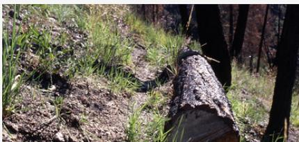
**Log barriers** are applied by anchoring felled and limbed trees into place on the contour of burned slopes to slow down water flow.
