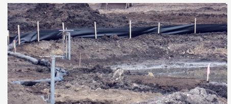
**Silt fences** are made of woven wire and fabric cloth anchored into place. They trap sediment from runoff in areas that are easy to monitor and maintain, such as flatter areas. They are not an effective solution for heavy sediment runoff and debris flows.
