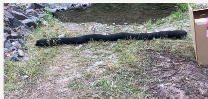
**Wattles**, either straw or wood, are used to slow and filter moving water on slopes, trapping loose sediment before it travels downslope.
