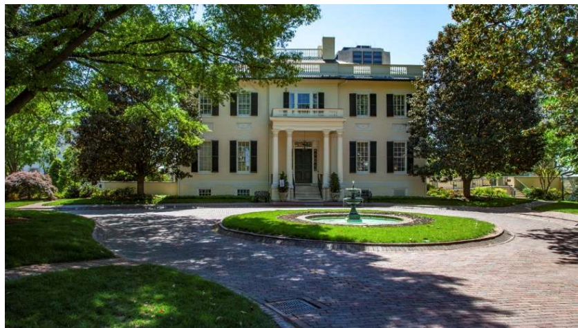
Virginia Executive Mansion — Exterior Facade | Richmond, Virginia | Federal / Neoclassical, 1813 | National Register of Historic Places
