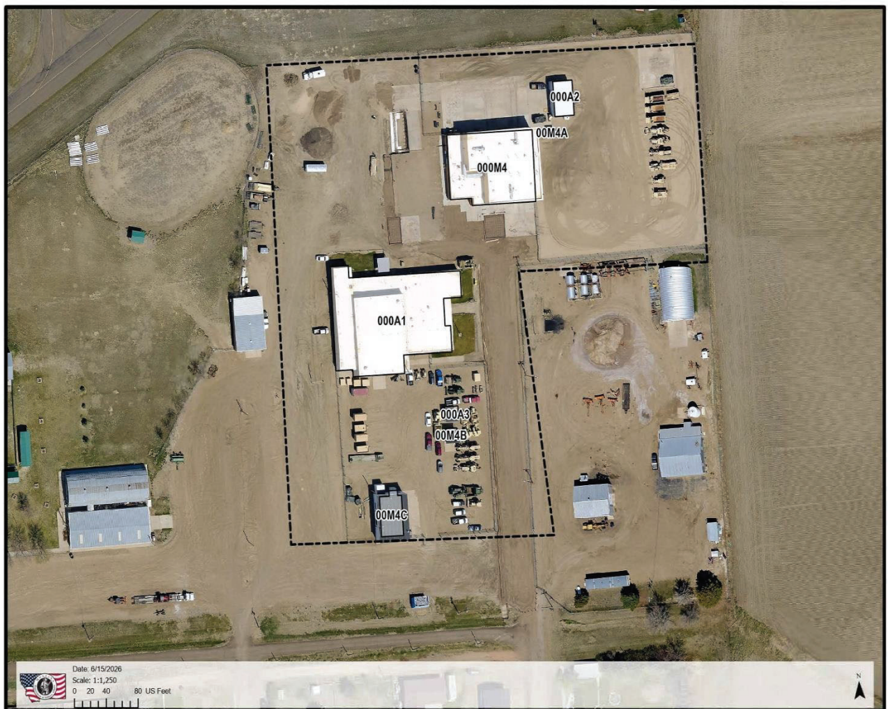
Culbertson Readiness Center and Vehicle Maintenance Shop
