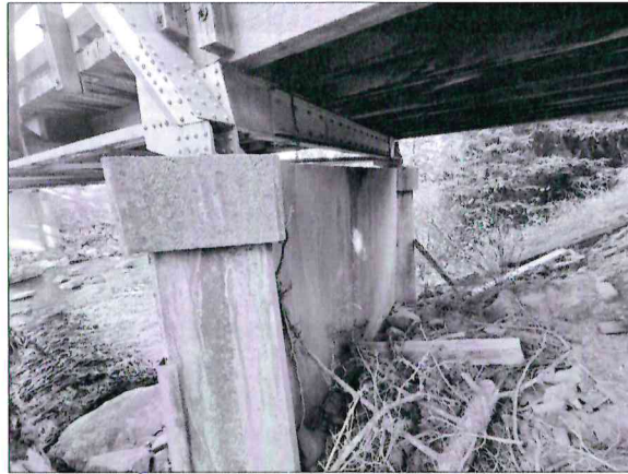
EXISTING BRIDGE PILES AND WINGWALL (EAST SIDE LOOKING DOWNSTREAM)
