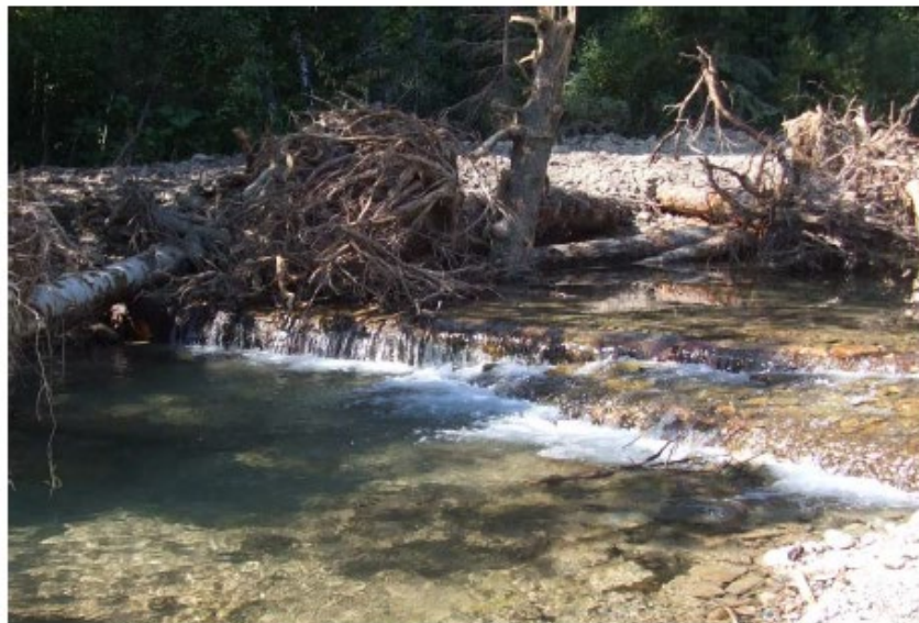
Figure C11. Example of a constructed cross log structure on the Cabinet Ranger District. C4 channel type.
