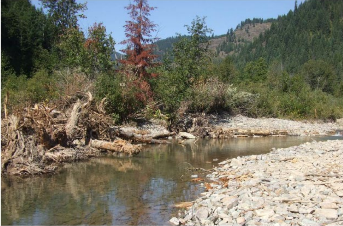
Figure C8. Example of a constructed log jam on the Cabinet Ranger District. C4 channel type
