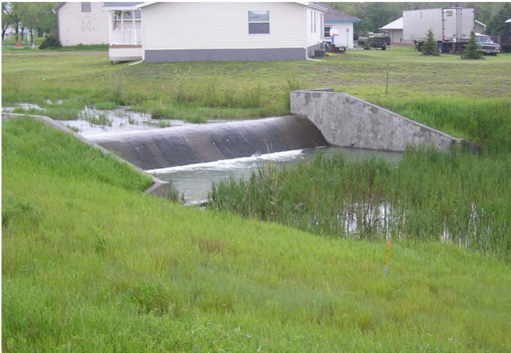
Drainage way below Baker Lake
