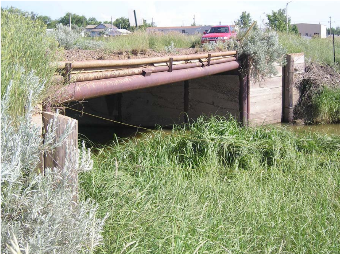
City Shop Bridge, Baker
