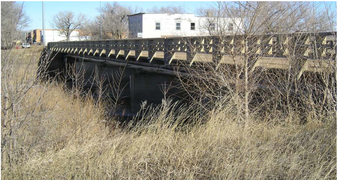
Highway 7 Bridge south edge of Wibaux
