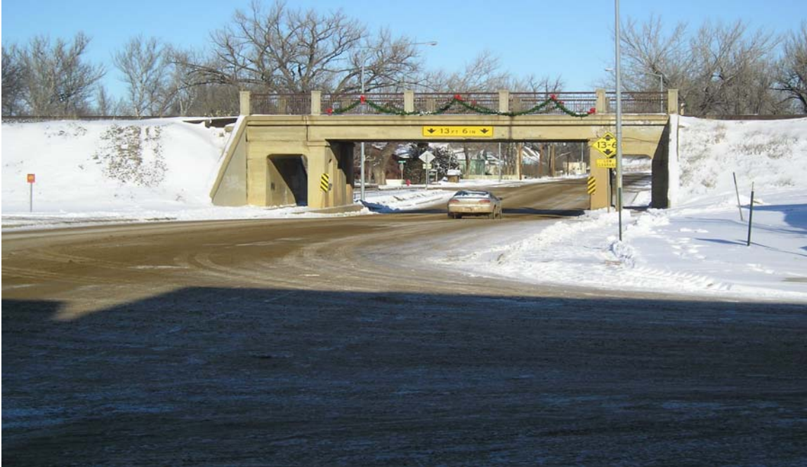
BNSF overpass located in the town of Wibaux
