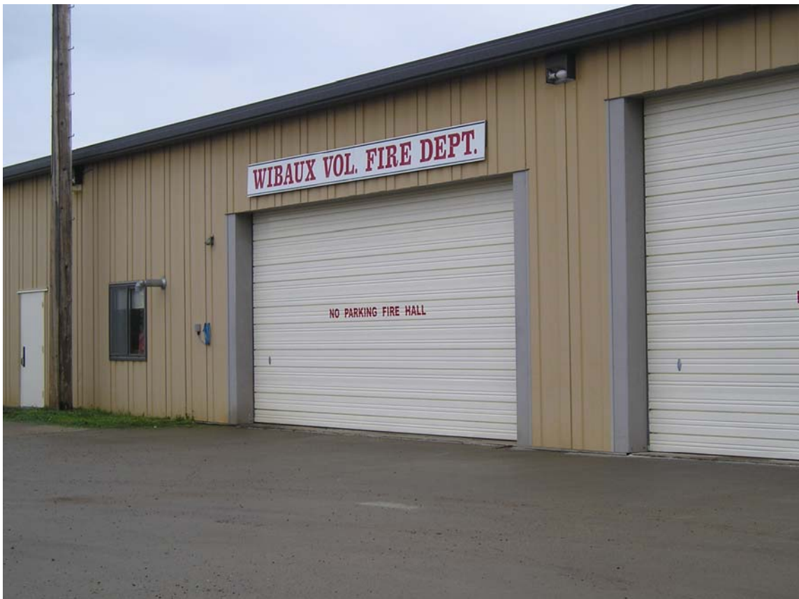
Wibaux Volunteer Fire Department Hall
