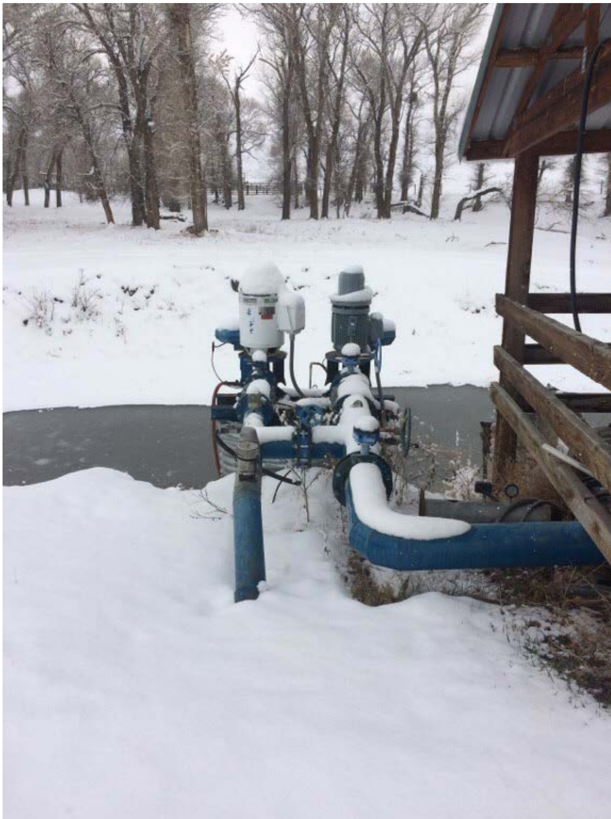
Figure 2: Pump site in the SW of Section 34, T6S R7E. Western pump (right pump in the picture below) supplies the full pivot in Section 34. The eastern pump (left pump in the picture below) supplies the remaining pivots and wheel lines.
