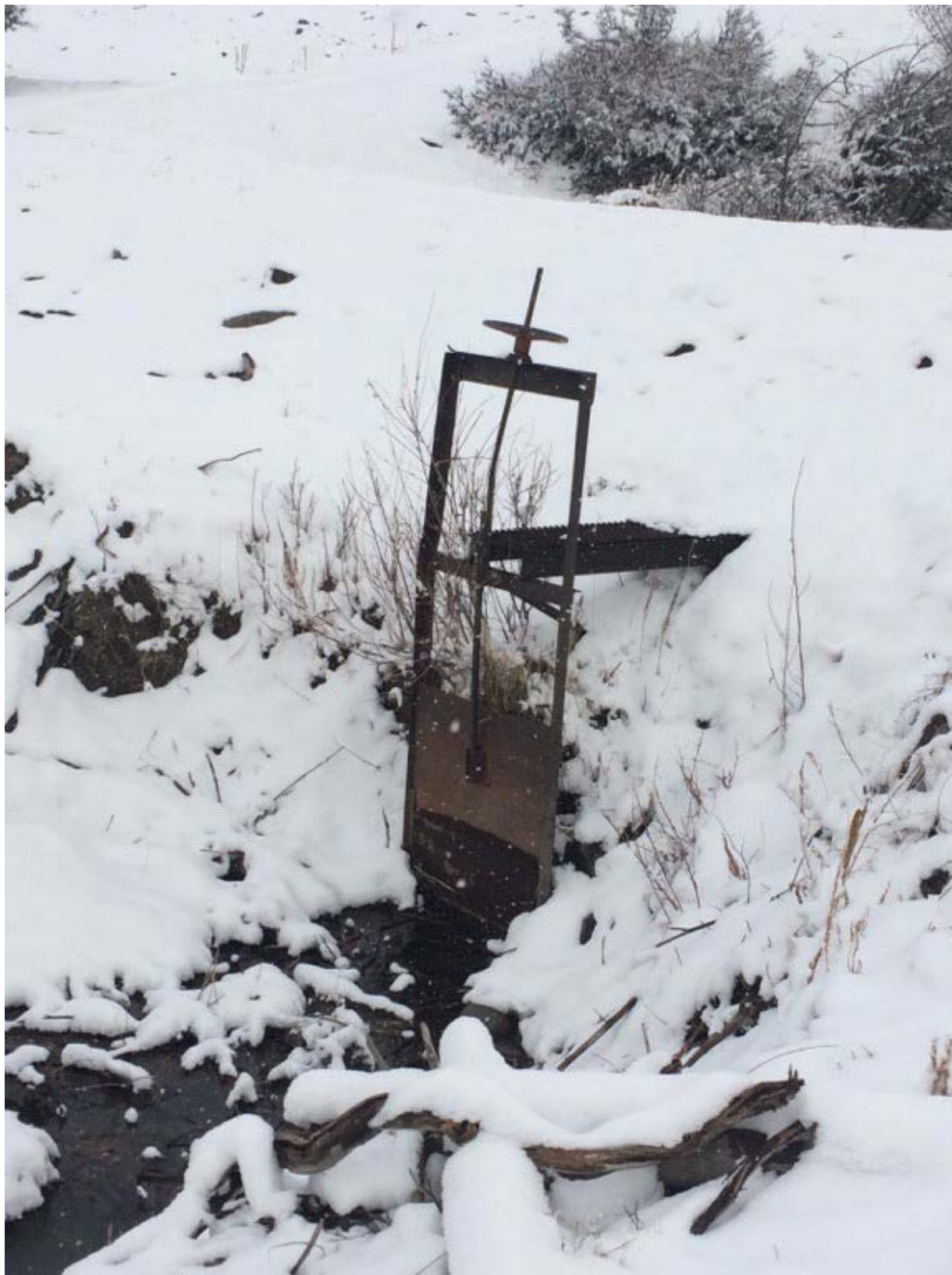
Figure 1: Stem and handwheel headgate at the Yellowstone River POD in the SW of Section 34, T6S R7E.
