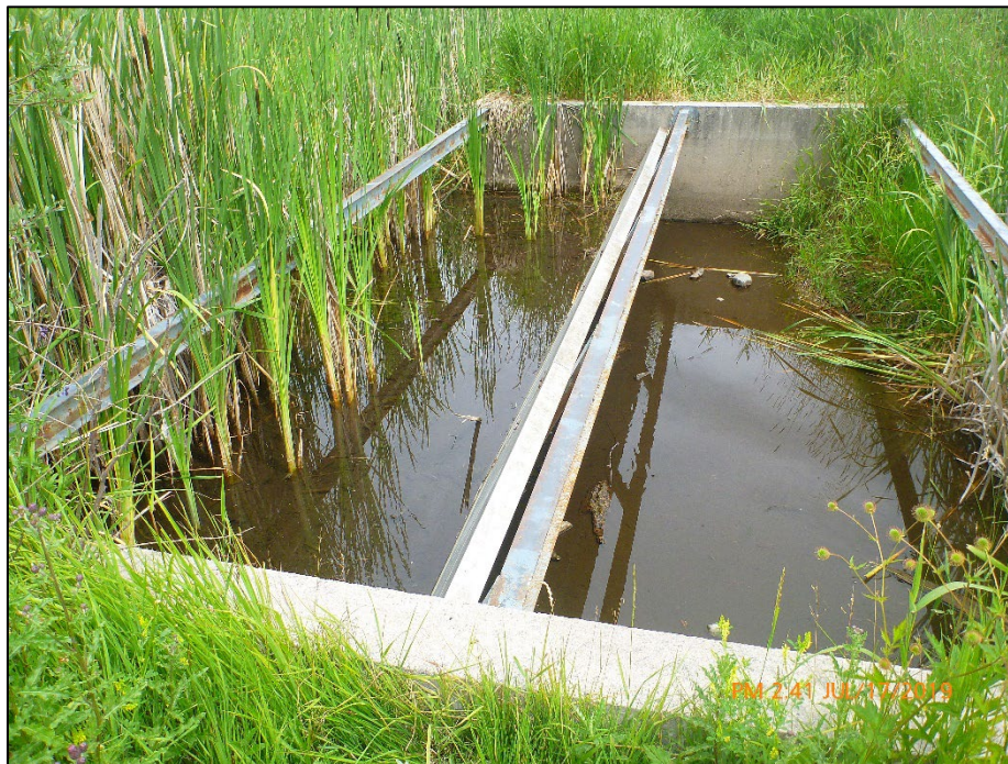
Figure 2: The weir structure that acts as an overflow structure for high lake levels.
