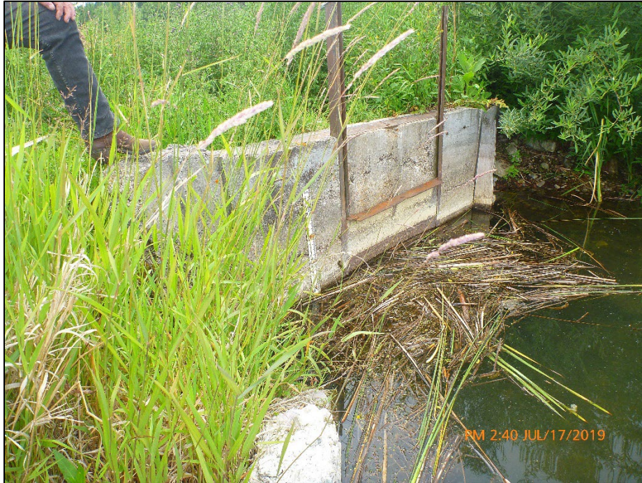
Figure 3: Headgate holding water in Lake Mary Ronan that allows the dam and headgate owner to release water into the CMP and into Ronan Creek on an unknown schedule.
