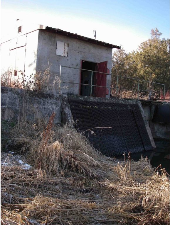
Photograph 32: Crow Pumping Plant building and intake structure.
