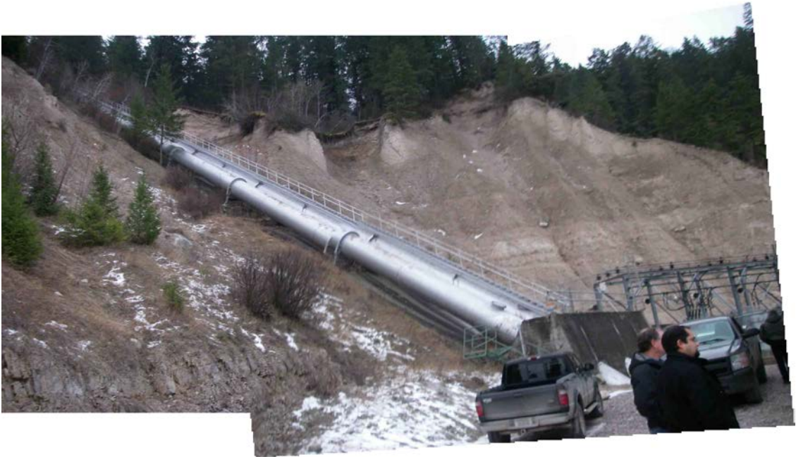
Photograph 3: Landslide area and three discharge penstocks for the Flathead Lake Pumping Plant.
