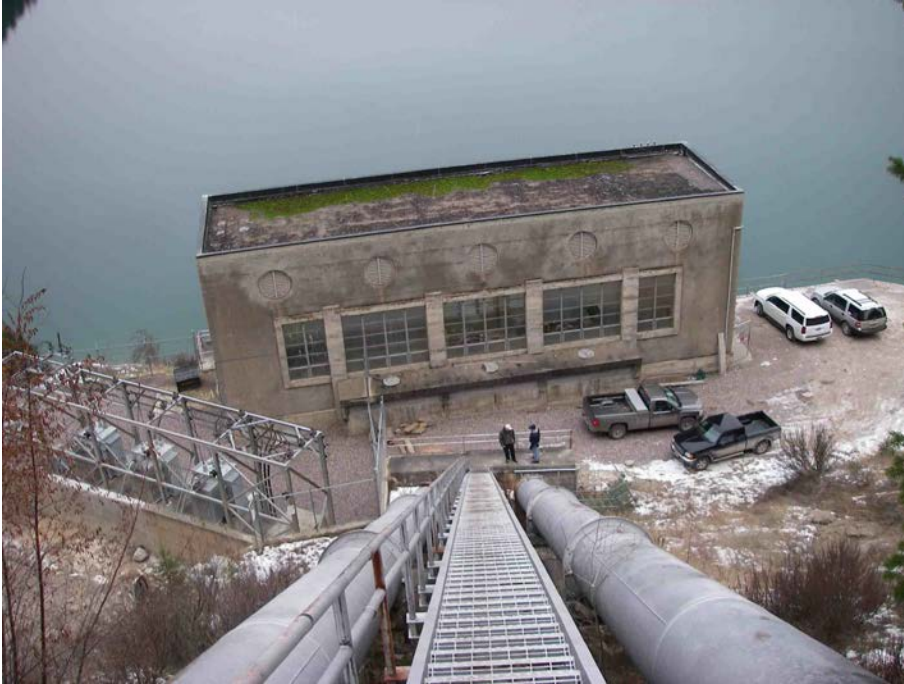
Photograph 6: Looking down the penstocks at the downstream side of the Flathead Lake Pumping Plant building.
