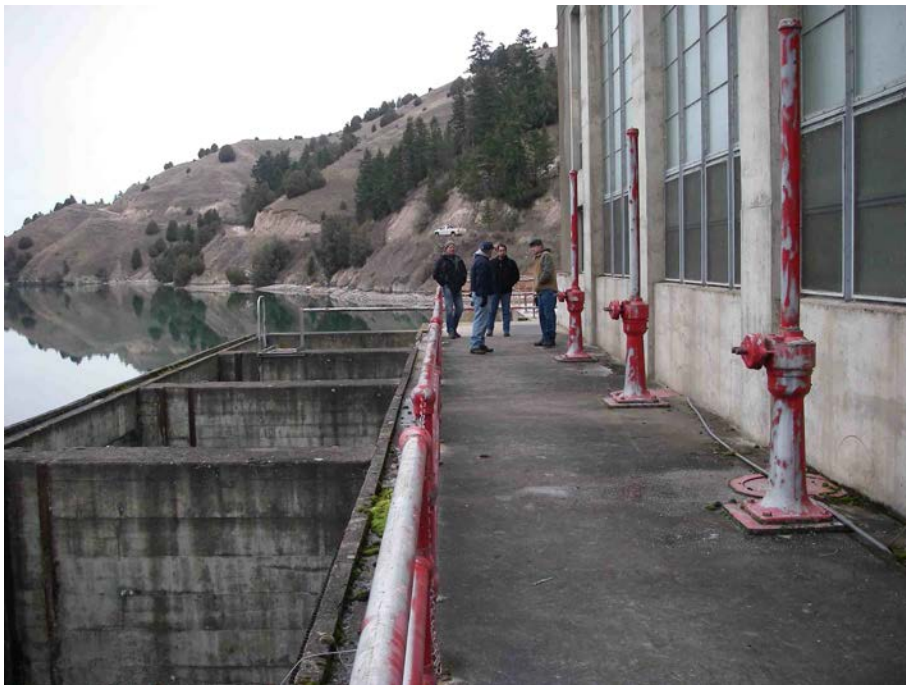
Photograph 4: Looking left across the top of the Flathead Lake Pumping Plant intake structure.
