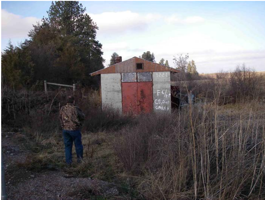
Photograph 31: Crow Pumping Plant building.
