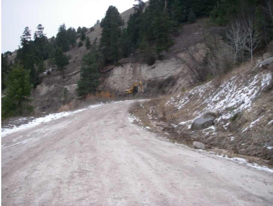
Photograph 7: Looking from the BIA Flathead Lake Pumping Plant along the access road at a landslide area next to the road.
