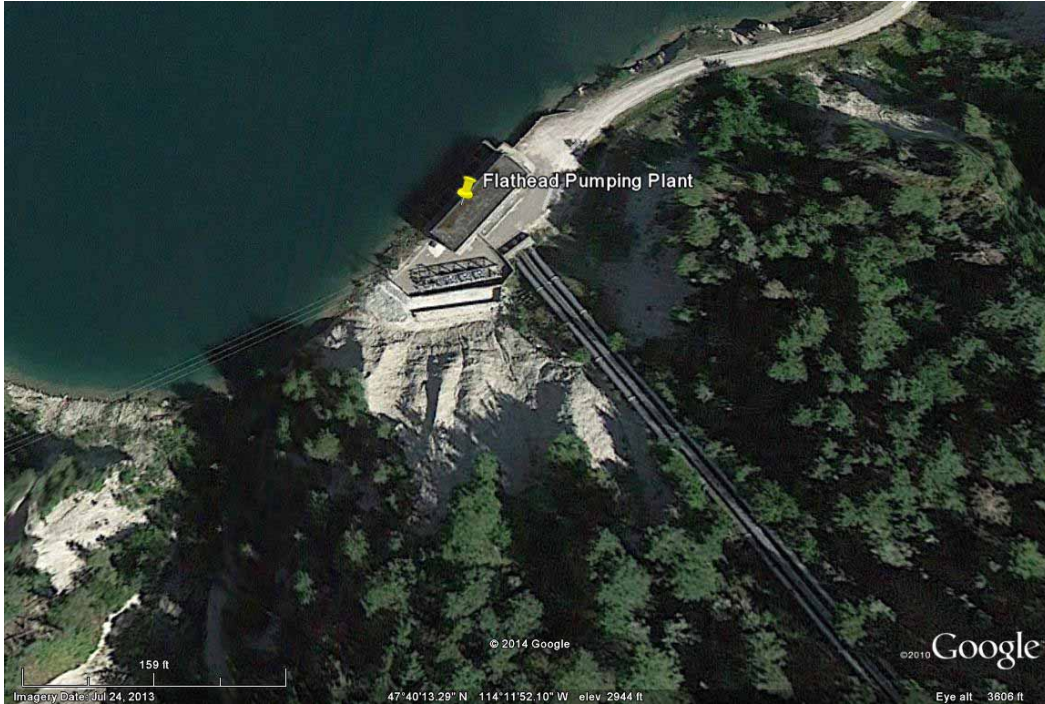
Photograph 1: Aerial photograph of Flathead Lake Pumping Plant showing the landslides on both sides of the three penstocks.
