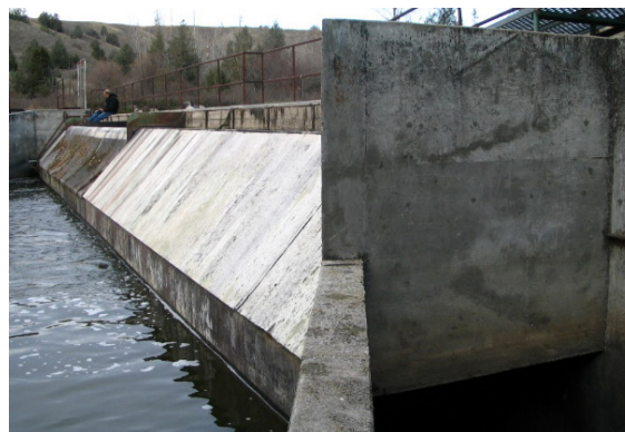
Figure 9. Downstream side of diversion dam in Crow Creek. Photo from HKM 2008 report (DD-12).
