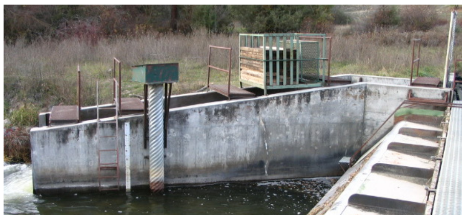
Figure 12. Fish ladder on the side of the diversion dam in Crow Creek. Photo from HKM 2008 report (DD-12).
