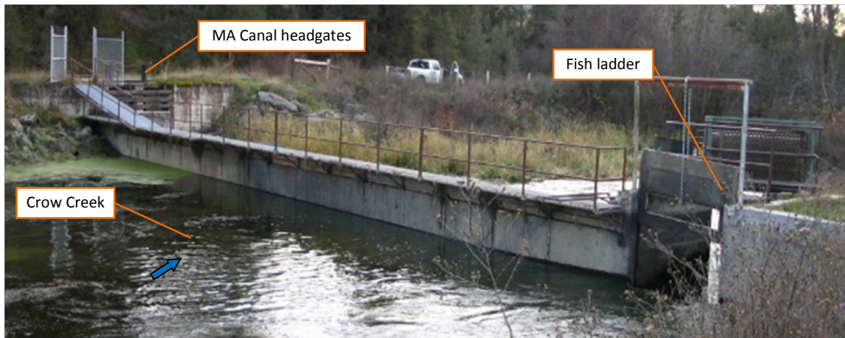
Figure 10. Upstream of diversion dam in Crow Creek for the MA Canal. Photo from HKM 2008 report (DD-12).
