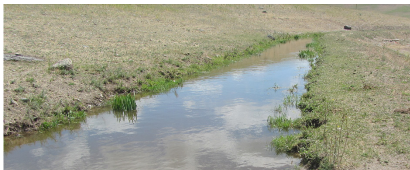
Figure 5. Example of the Hillside Ditch with little freeboard
