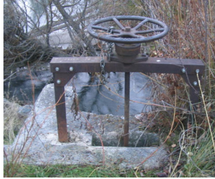
Figure 5. Existing Mission H Canal headgate. Photo from HKM 2008 report (HG-55).
