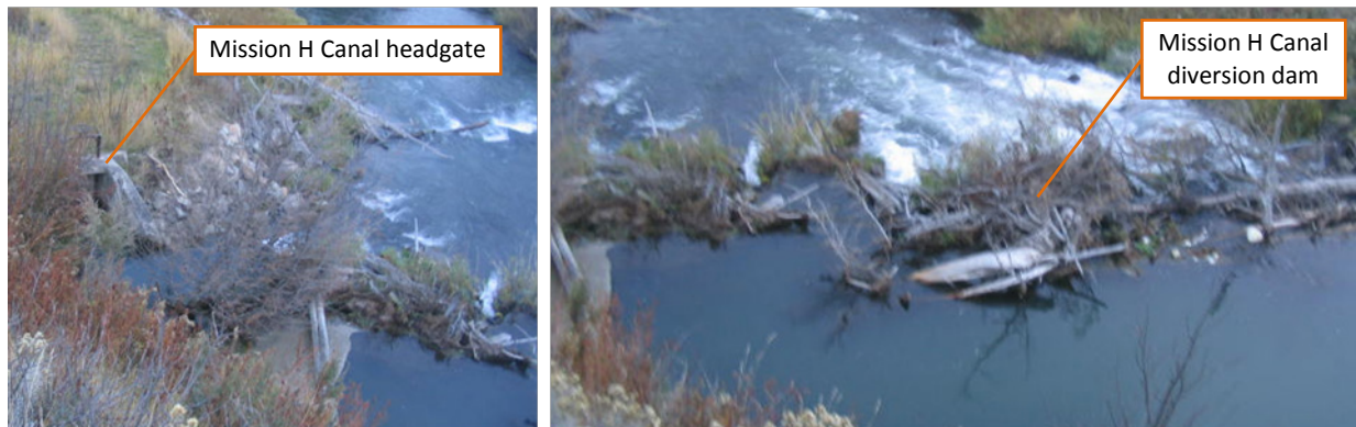
Figure 4. Existing Mission H Canal diversion on Mission Creek. Photos from HKM 2008 report (HG-55).
