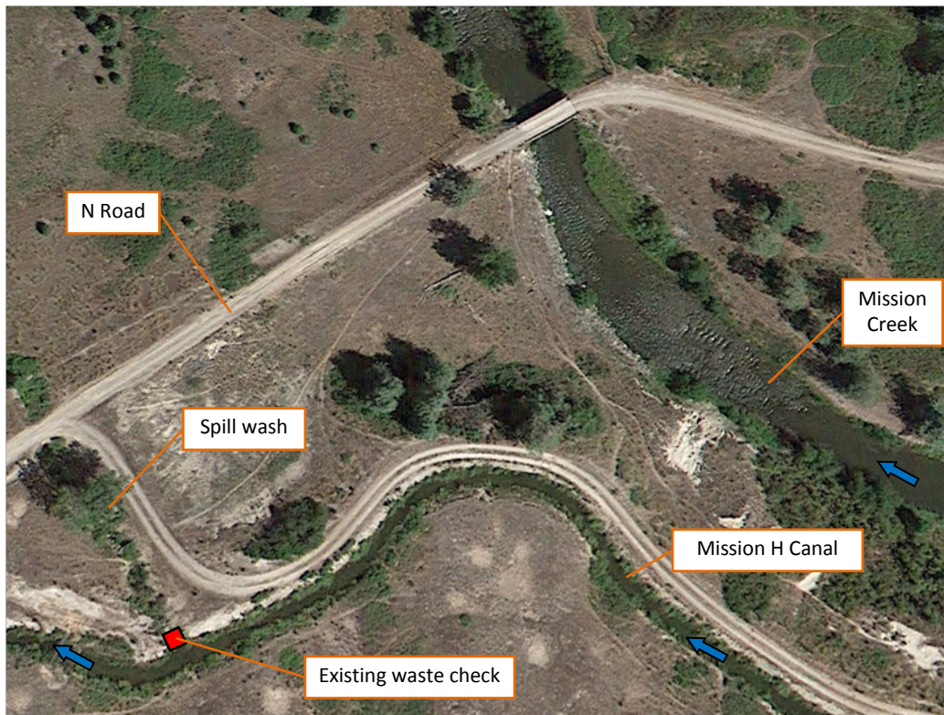
Figure 7. Mission H Canal at the existing waste check structure located approximately 1.3 miles downstream from the canal diversion
