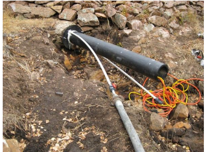
Photo 3: Grouting HDPE Liner pipe. 3
