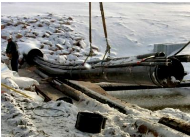
Photo 2: Installing HDPE Liner pipe. 2
