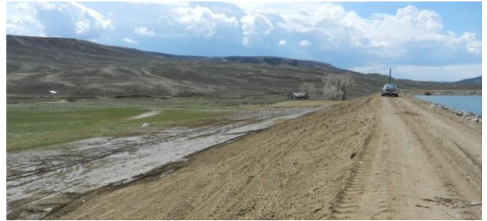
Figure 1. Disperse Seepage at Dam Toe (Wyoming NRCS)
