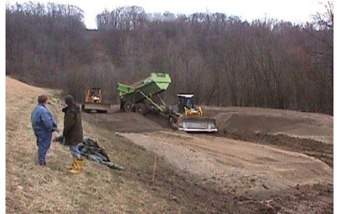
Figure 3. Inverted Filter Berm at Salt Fork Dam [4].
