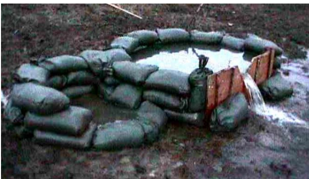
Figure 7. A Sandbag Ring with V-Notch Weir [4].
