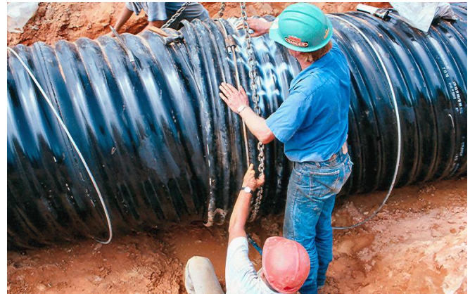
Figure 1. A CMP Conduit Being Installed [1].
