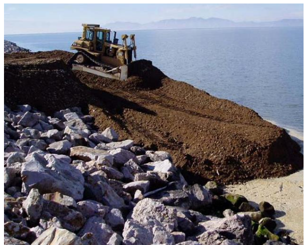
Figure 6. A Placement of Upstream Berm at AV Watkins Dam [4].
