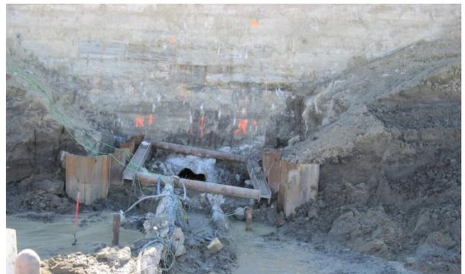
Figure 2 - Uncontrolled downstream seepage exiting with reservoir down to deadpool, rehabilitation of headworks, Lake Frances Dam, MT (Note pin boils near toe; the two wells were ineffective). (Courtesy of Montana Department of Natural Resources and Conservation)
