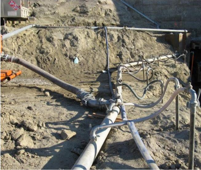
Figure 5 - Wellpoint system along trench excavation, Lake Frances Dam Outlet Works Rehabilitation, MT (Courtesy Montana Department of Natural Resources and Conservation)
