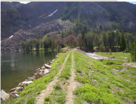
Noble Lake Dam, Madison County
