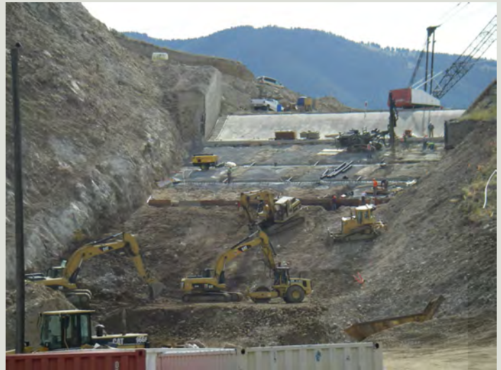
Ruby Dam spillway under construction, Madison County
