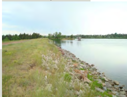
Castle Rock Reservoir Dam, Rosebud County
