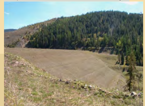
Kootenai Development Impoundment Dam, Lincoln County
