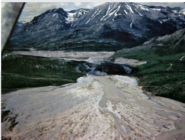
1964 Swift Dam failure, Pondera County
