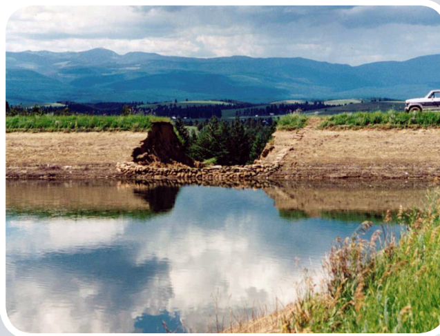
Eureka Dam Failure
