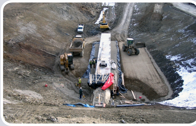
Construction Work on Deadman's Basin Dam
