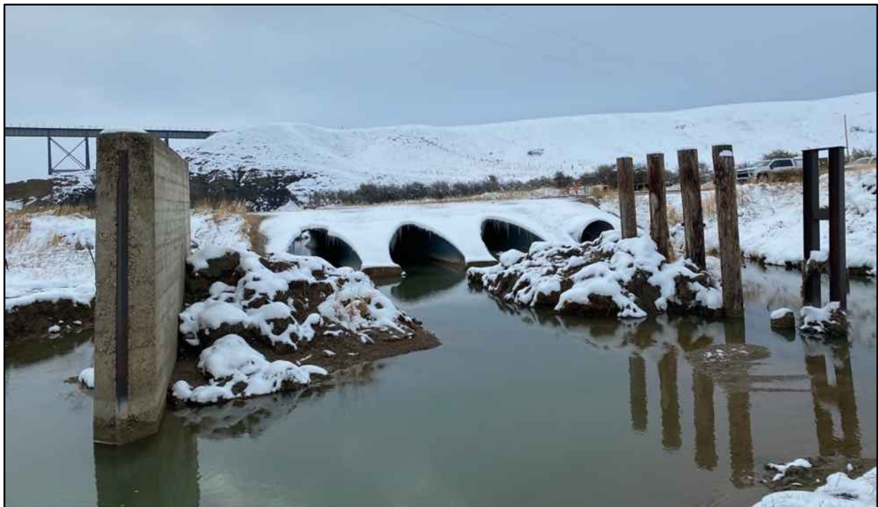
Figure 7: Upstream Face of Structure MUD_020_GPS with Historic Bridge Bents
