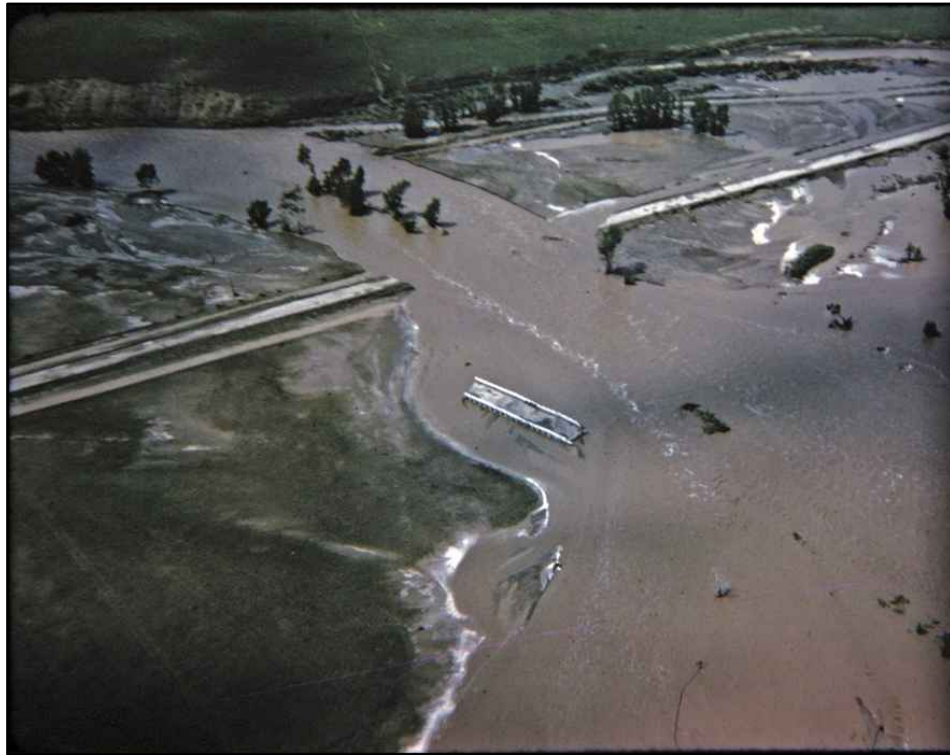
Figure 6: 1964 Flood Photo on Deep Creek, Hwy 287 (Structure DEE_020_SI)
