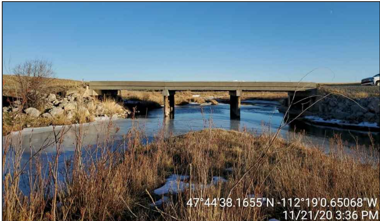
Figure 12: Pishkun Road Bridge (WIL_030_SI) Over Willow Creek
