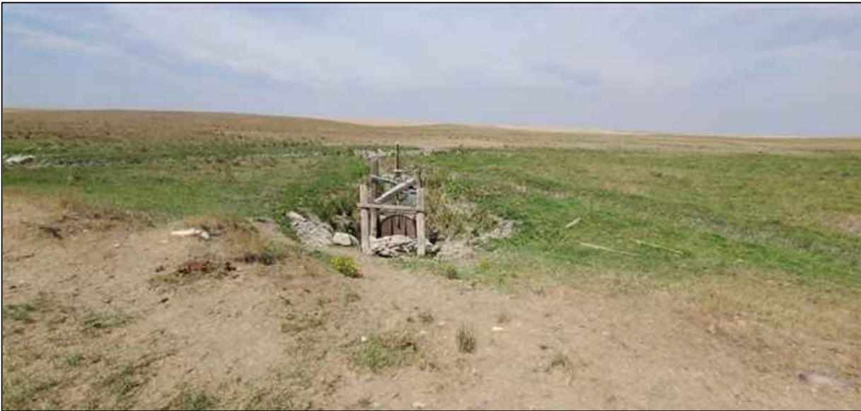
Figure 17: Closed Check Structure on Foster Creek Reach FC-2
