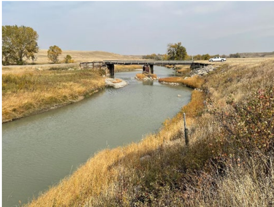
Figure 10 - Bridge TET_030 (20 th Lane NE) Looking Downstream from Streamflow Measuring Station
