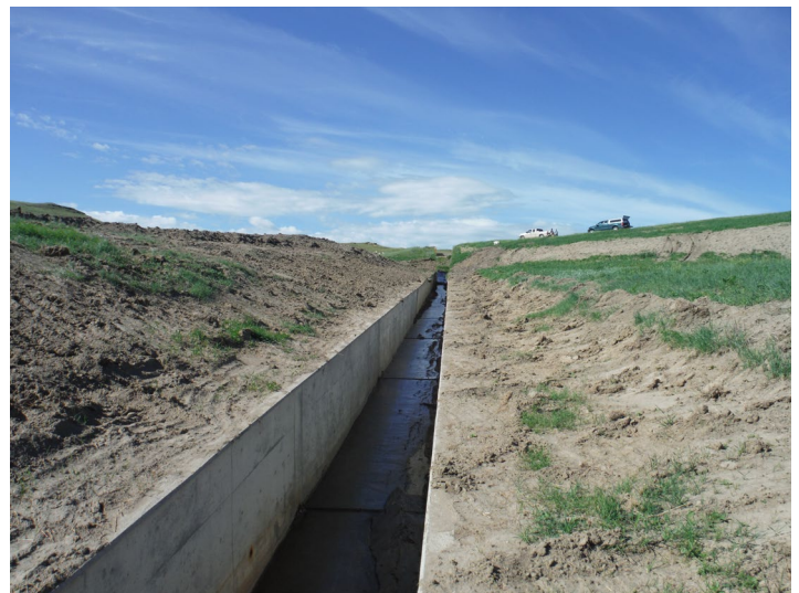
Spillway Chute at East Dam
