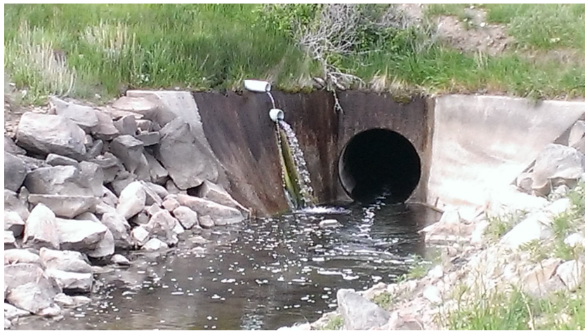
Outlet at North Dam
