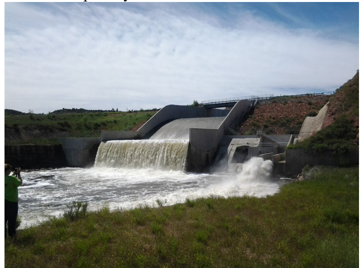
Outlet and spillway
