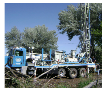
Ron Askin Drilling, Miles City MT
