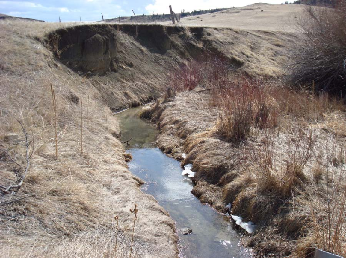
Grove Creek above culvert under Grove Creek Road: March 24, 2008
