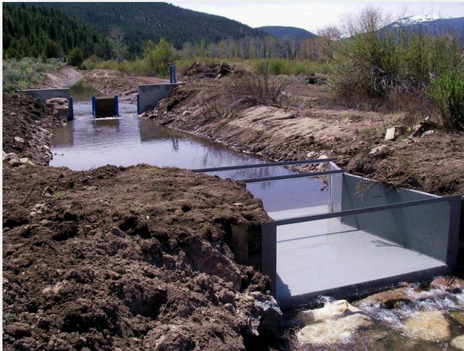
Figure 14: Upper PKR Ditch improvements include a Cutthroat Flume and a screw-gate turnout at Swamp Creek. (photo by D. Amman)
