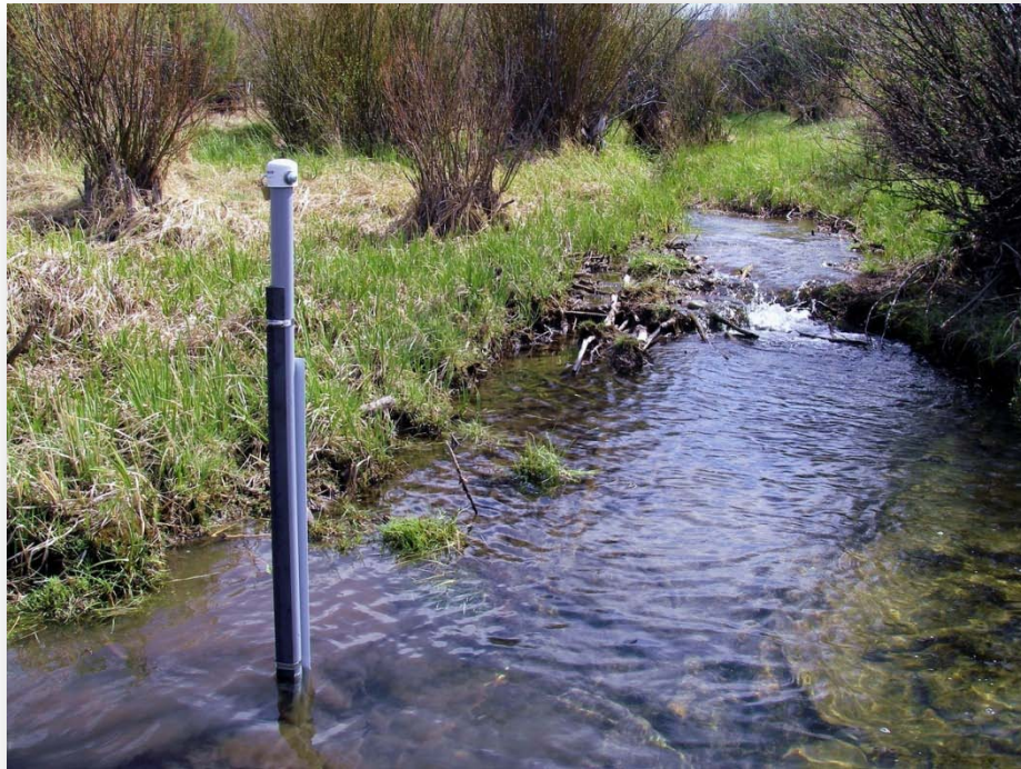
Figure 1: TruTrack water level recorder installed in Smart Creek
